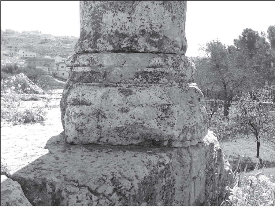
4. Profile of the bases: southernmost of the three bases in the mausoleum showing the scheme of the Ionic base (so-called Attic version with two tori , a trochilos between them and two listels).
